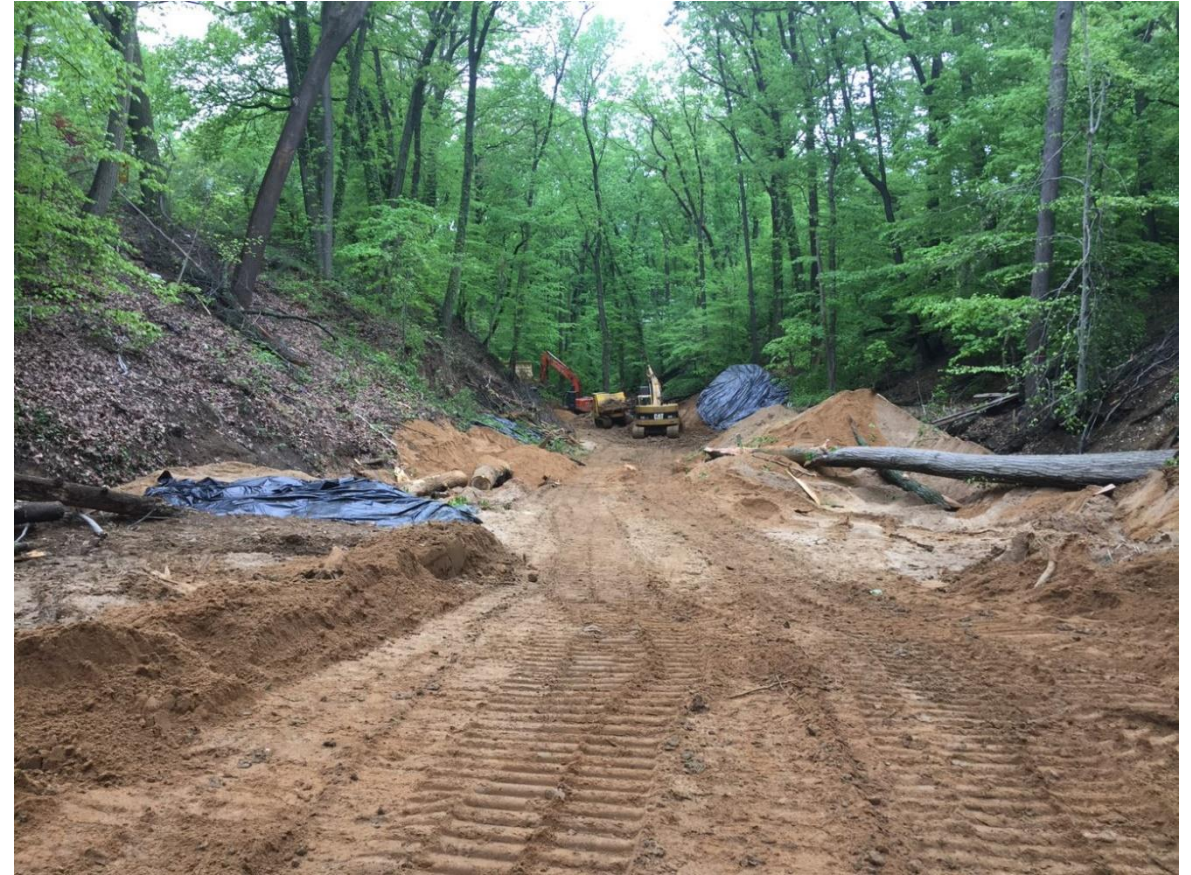
Connecting to floodplain Pools for habitat & to dissipate energy
