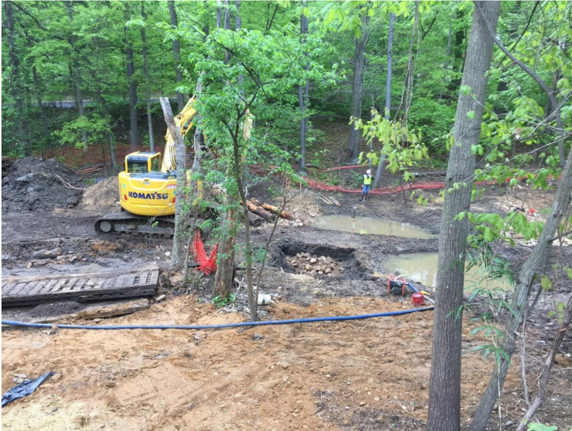
Filling the incised channel Buried logs in floodprone areas
