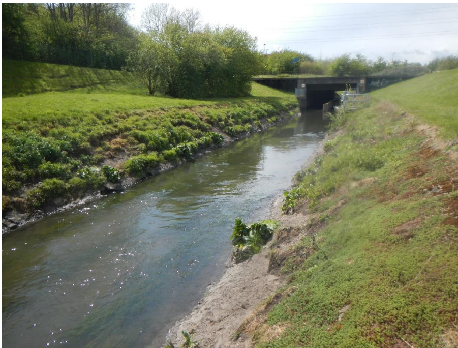
Figure 3: Photo of the sampling site at King's Meadow (site 10). This site is the most heavily modified of those sampled; the river is straightened and over-deep, the bed and banks are reinforced with concrete, and there are several outfalls and bridges. This means overall habitat diversity is limited which restricts the ecological quality of the site.
