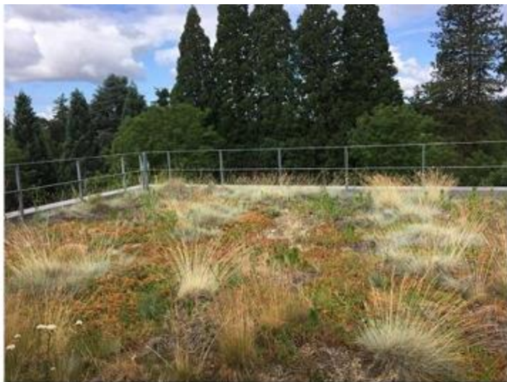
Green roof / ecoroof
